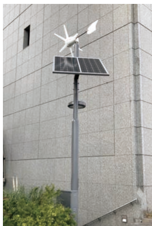
Installation of solar-wind streetlights (Daiwa River Gate)
