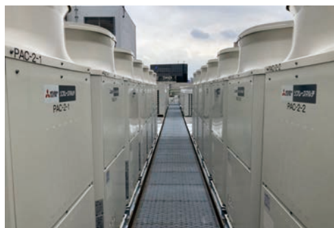
Implementation of upgrading to zoned air-conditioning (Daiwa Ginza)
