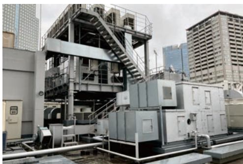
Upgrading of air-conditioning equipment (Daiwa Akasaka)
