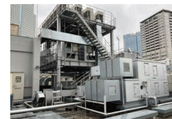
Upgrading of air-conditioning equipment (Daiwa Akasaka)
