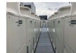
Upgrading of air-conditioning equipment (Daiwa Ginza)
