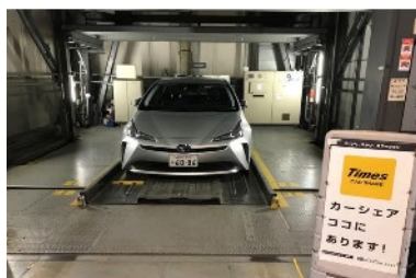
Installation of car sharing port (E SPACE TOWER)
