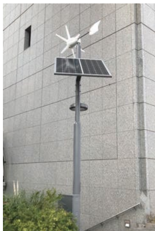
Installation of solar-wind streetlights (Daiwa River Gate)
