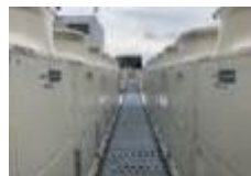
Renewal of air-conditioning equipment (Daiwa Ginza)
