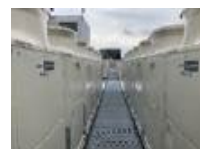
Renewal of air-conditioning equipment (Daiwa Ginza)
