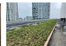
Rooftop garden (CONCURRED Yokohama)
