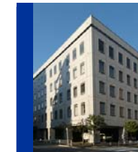
Shuwa Tsukishima Bldg.
